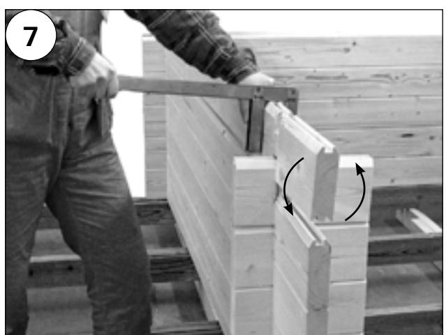
**EN** **Figure 8.** After laying 4–9 rounds of logs, install the front door. Knock the frame downwards from both upper corners to make sure that the frame is correctly positioned.
